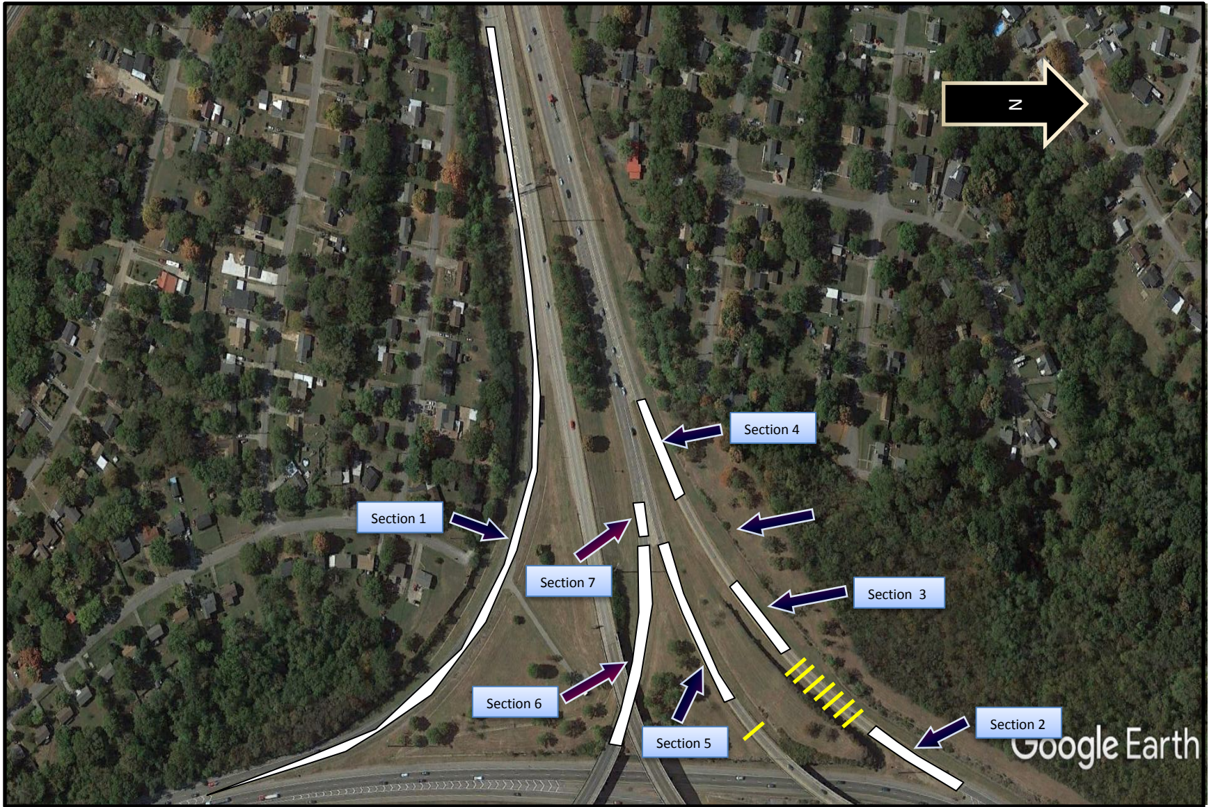
Figure 10: I24 and I40 Interchange
